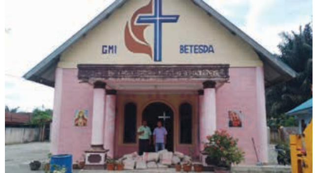
GMI Betesda Church Renovation – Rubber Hock Lie Donated 30 Sacks of Cement
