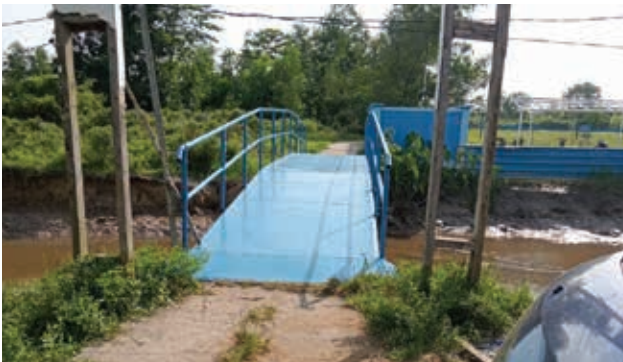
Assisting to Repair Bridges and Local Health Facilities – Hok Tong Keramasan's Concern for Workers and Local Communities
